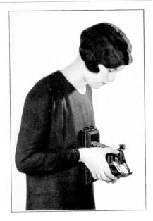
When making instantaneous exposures or snapshots with any Kodak, hold it firmly against the body as shown; or against the face if using the metal frame finder. When pressing the exposure lever, hold the breath for the instant. If the Kodak is moved during the exposure, the picture will be blurred.
